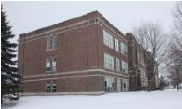
View from the Northwest
