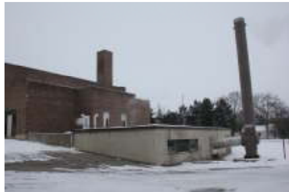
View from the Southeast
