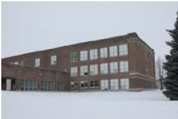
View from the Northeast
