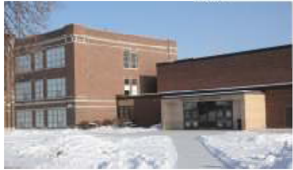
View from the Southwest
